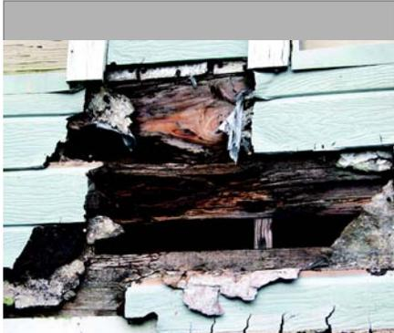
**Wood decay is different from termite damage; however, they can occur together.**
