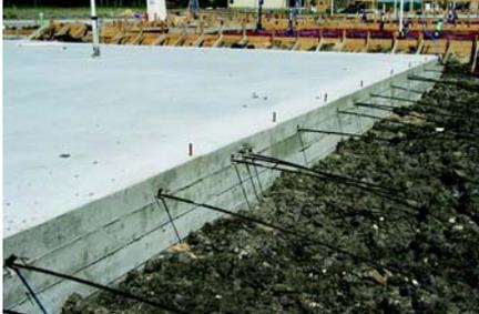
**A post-tension monolithic slab.**
