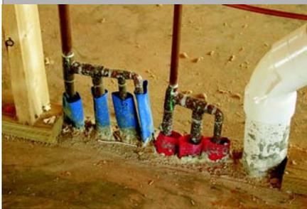
**Termites can penetrate a home where pipes enter at a slab.**
