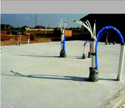
**Termites can enter at plumbing penetrations in the slab.**
