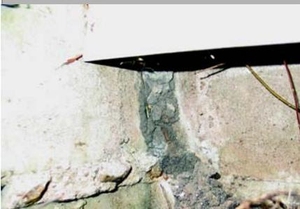
Example of termite mud tubing partially hidden in a foundation corner.
