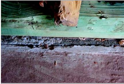
**A joint between the foundation wall and basement where termites can enter.**
