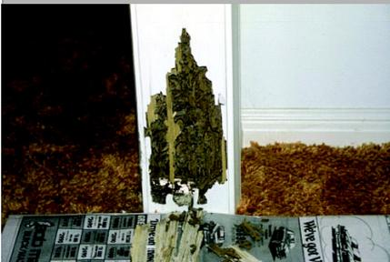
An example of termite damage in a home just beneath a normal looking surface.
