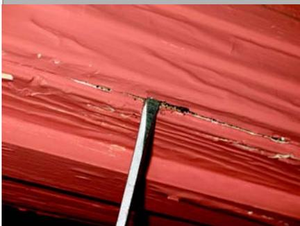
**A technician uses a screwdriver to probe wood for termite evidence.**
