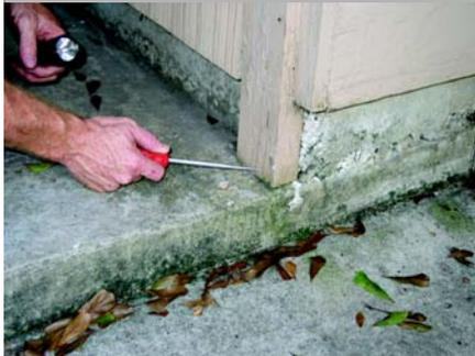
**Wherever wood meets the slab or the ground is a likely entryway for termites. Probing with a screwdriver can help detect hollow wood where termites have tunneled.**
