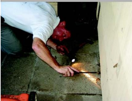
A termite inspector looks for evidence of termites where siding obscures the foundation.
