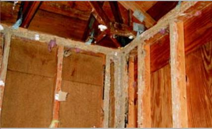
Proper inspections are a must. Termites can cause thousands of dollars of damage without detection, like hidden damage behind walls as shown above.
